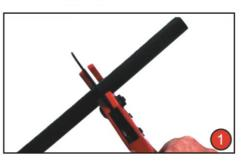
Using pipe cutter to cut the pipe squarely and ensure it is clear of burrs.
